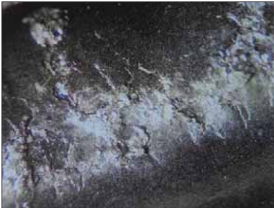
Raceway with Cracks and Pits
